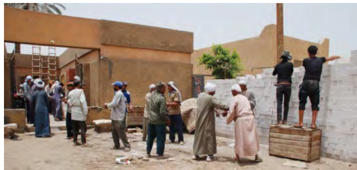
Photo 29. Transferring the remaining unused bricks to the store.
