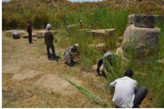
Photos 2b. Cleaning work
